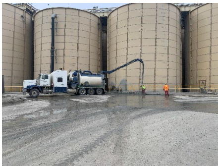
Figure 3. Spill clean up photograph (Jan 31)
