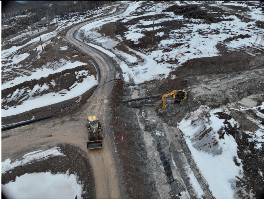
Figure 17. Cleanup progress (Feb 7)
