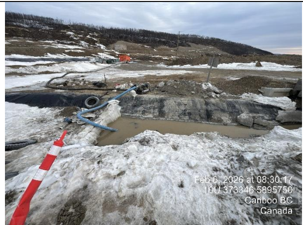
Figure 15. Cleanup progress (Feb 6)
