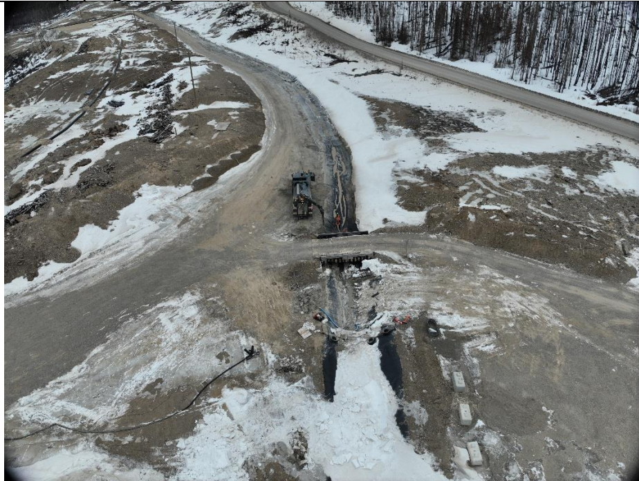
Figure 18. Cleanup progress (Feb 11)
