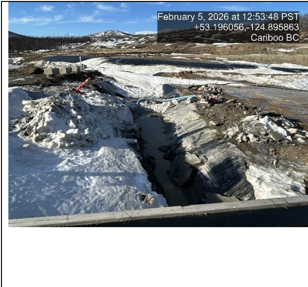
Figure 10. Cleanup progress (Feb 5)
