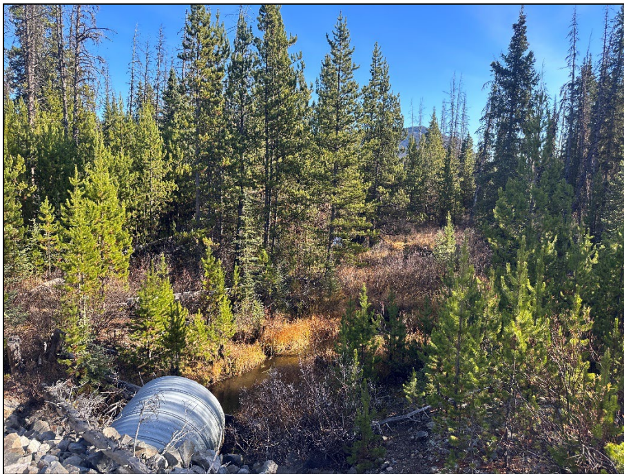
Plate 4.4-2. Large functional culvert on Van Tine Creek with intact riparian vegetation on both sides.
