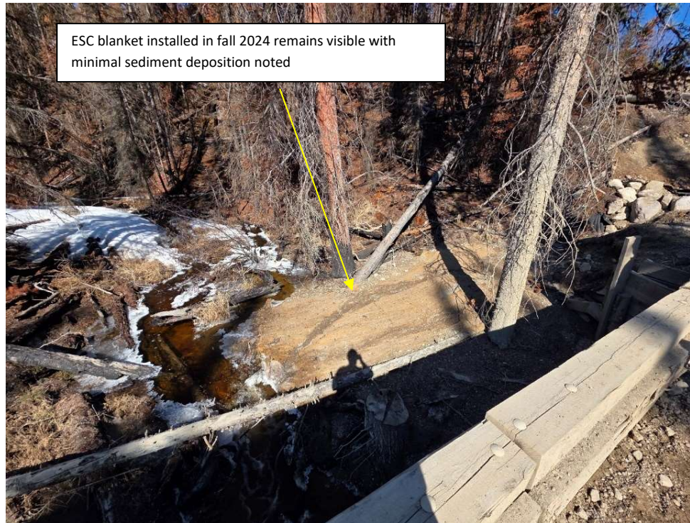
Photo 113555-10. Overview of base of C-trail access road drainage ditch adjacent to Watercourse 636 after spring melt period. Sediment transport into watercourse observed to be minor at time of visit.
