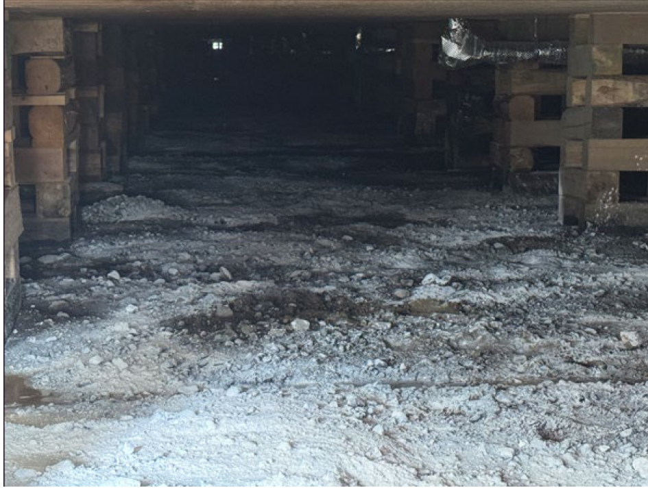
Photo 6: Spill Clean Up
