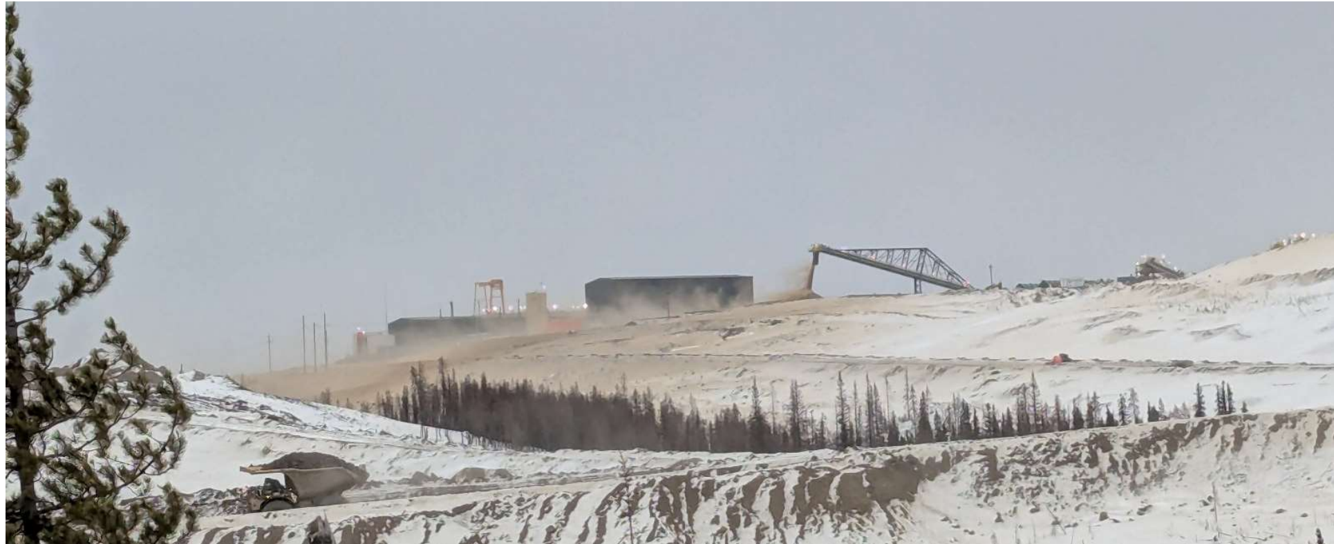
Photo 113363-5. Overview of high-grade ore dust generation from conveyor drop point at the Plant Site on March 19, 2025.
