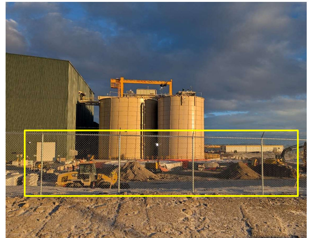
Photo 114726-1. Plant site updates associated with the Phase 1A expansion continue.
