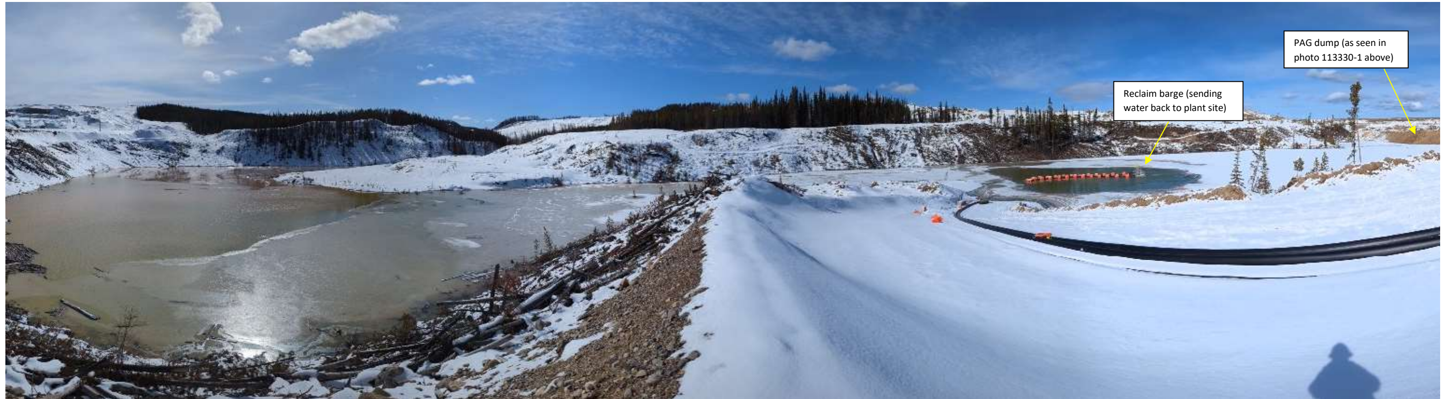
Photo 113323-2. Overview of lower portion of the Tailings Storage Facility. Water levels continue to increase and back up into the former Davidson Creek valley (left side of photo).
