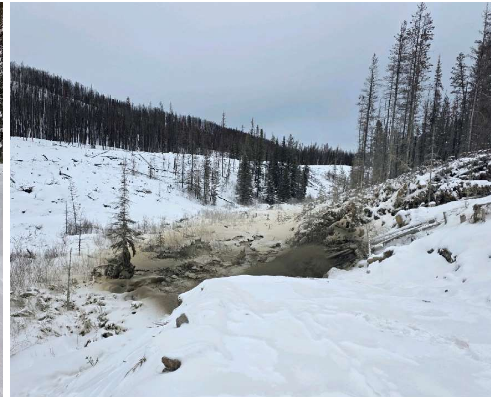
Photo 113133-1. Tailings pipeline discharge point into the upstream end of the TSF.
