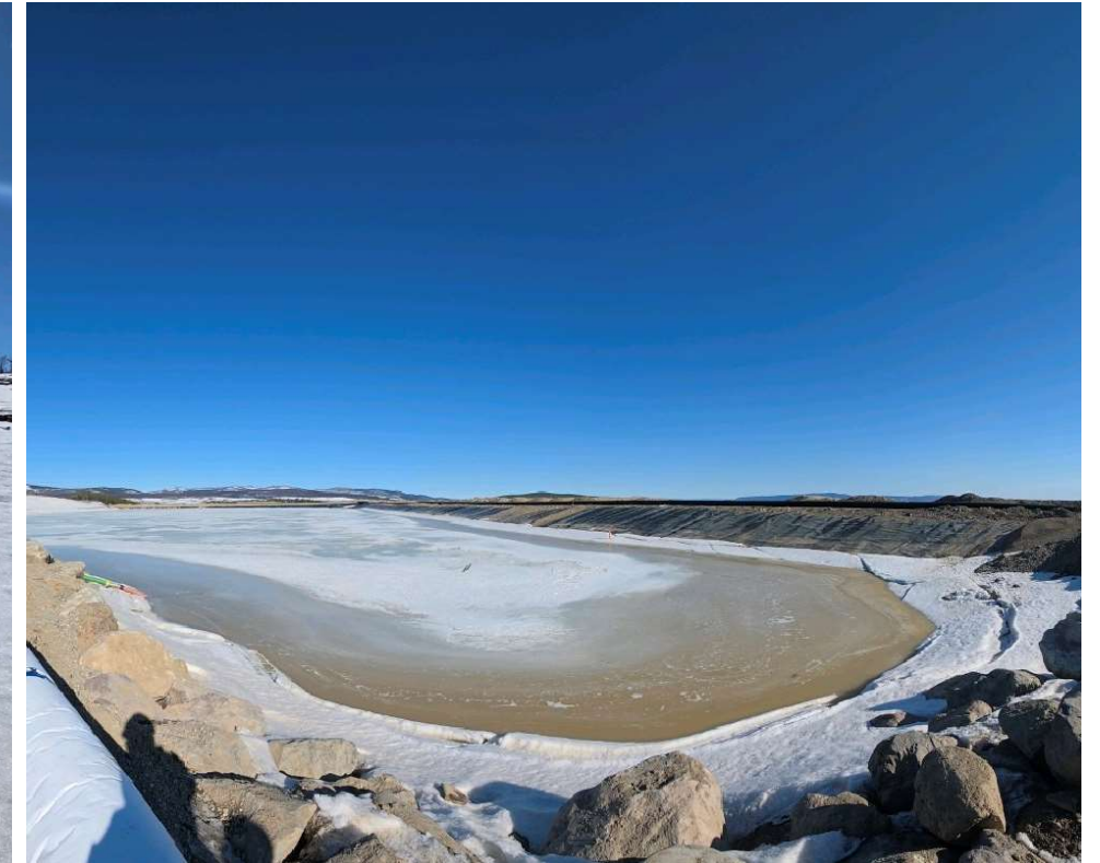
Photo 113550-1. Overview of a portion of the WMP. The IEM understands BWG continue to have issues with the turbidity of the water within the pond and are currently reviewing options for treatment.
