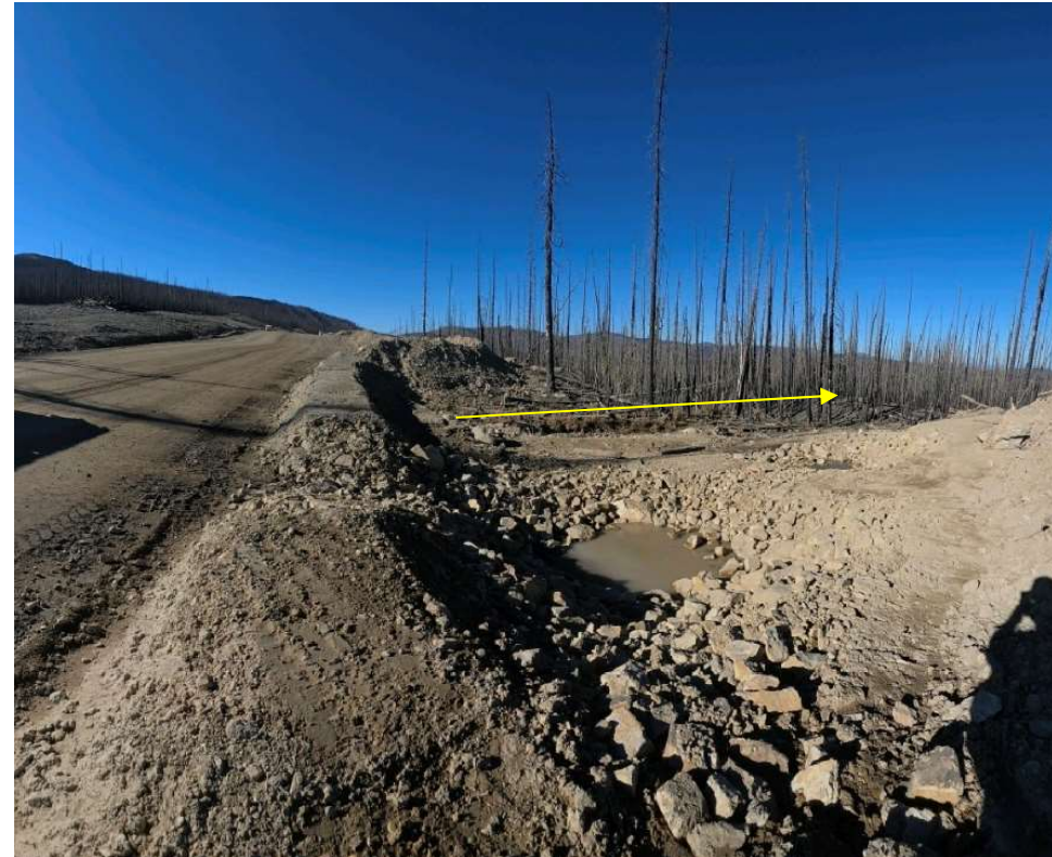
Photo 114455-1. Example of a collection sump installed within the ditch line along the road to the explosive magazine area. Area has connectivity to tributary to Mine Creek. Approximate flow pathway towards tributary indicated on photo.
