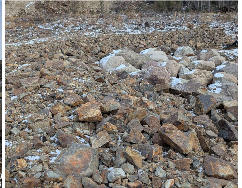
Photo 114723-1. Riprap placed at the IECD emergency overflow channel.
