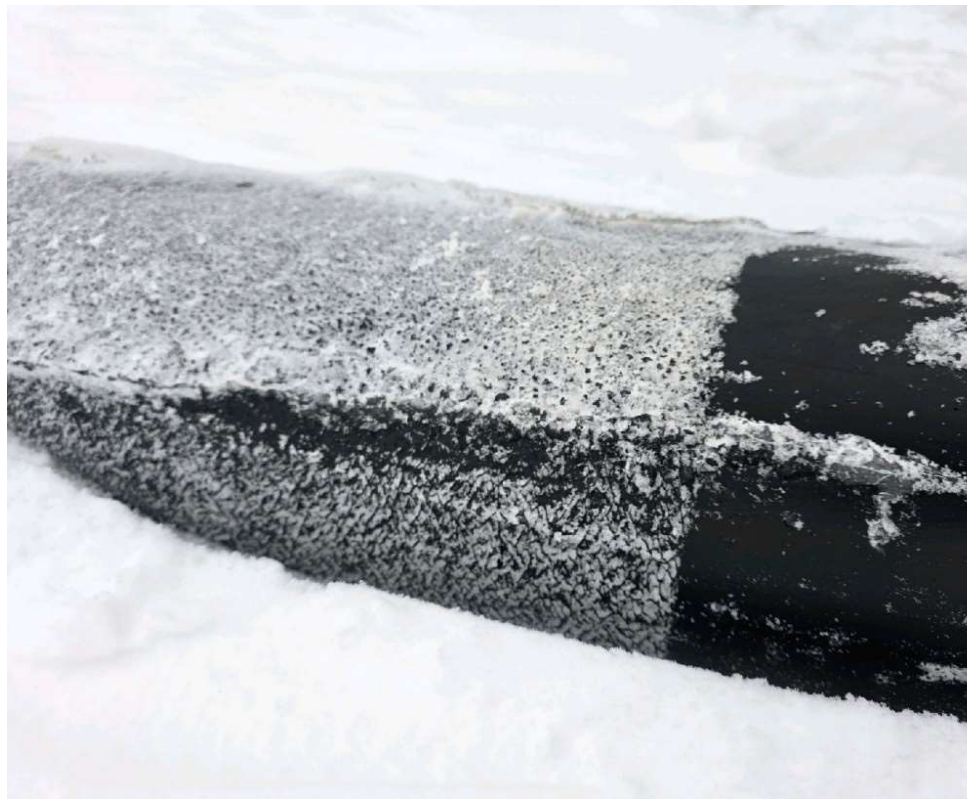
Photo 113124-3. Textured liner installed within the LGO stockpile pond.
