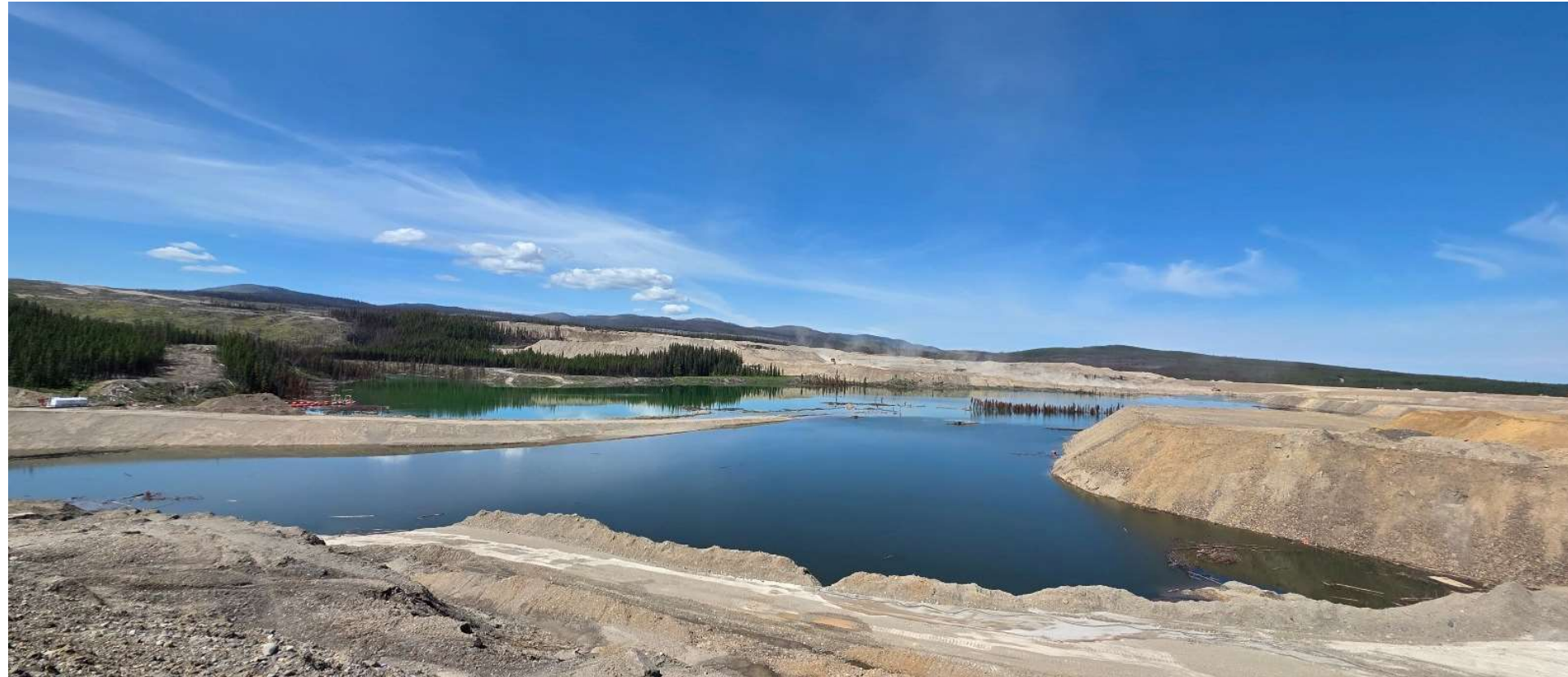
Photo 114075-2. Overview of the Tailings Storage Facility facing towards the TSF dam.
