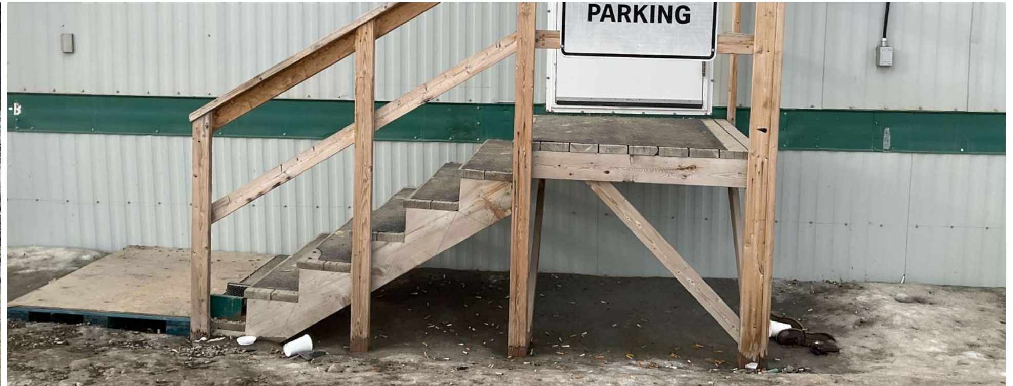
Photo 112960-2. Example of domestic waste (food/cigarette butts) observed outside of entrance to bunk at the Construction Camp. BWG has confirmed the area was cleaned up.
