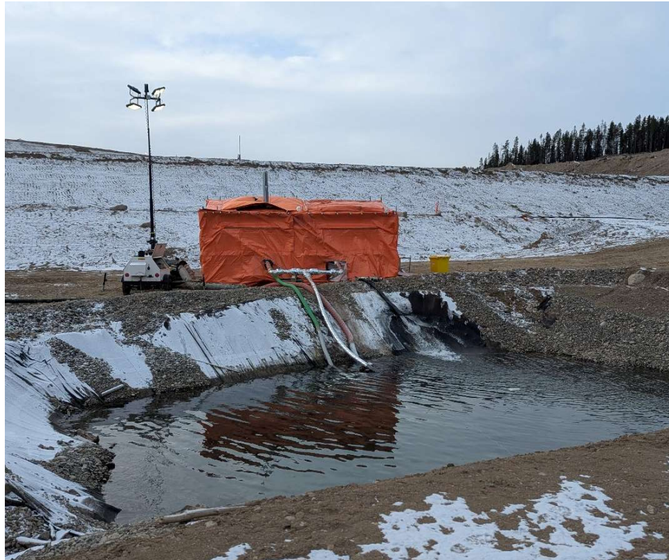
Photo 114712-5. Photo of the IECD sump capturing groundwater downstream of the IECD. WAD cyanide has been detected in groundwater at this location. BWG currently pumping water back upstream to the IECD and TSF.
