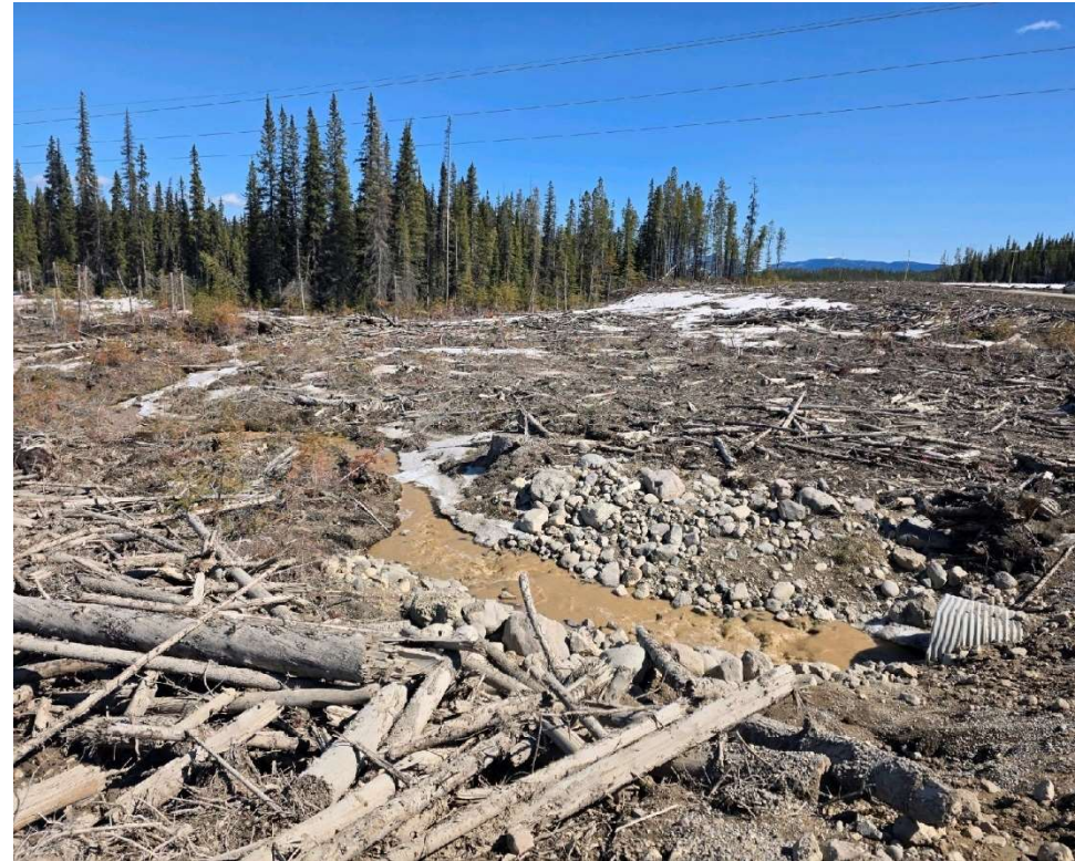
Photo 113513-10. Turbid flow in Watercourse 146 (fish salvaged) sourced from roadside ditches (see Photo 113513-9). Photo taken morning of April 15, 2025.
