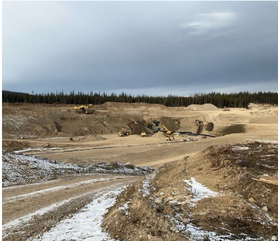
Photo 114704-2. Crews working on the western side of the Fresh Water Reservoir.
