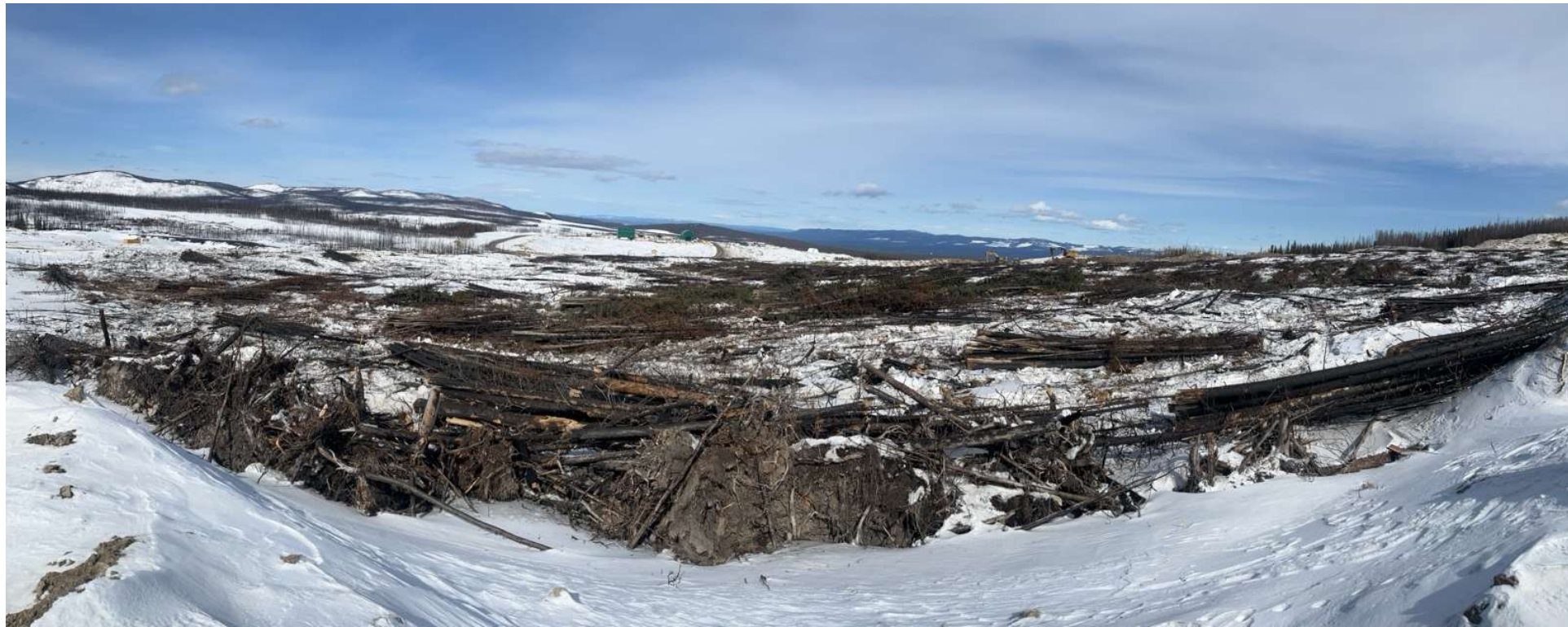
Photo 113324-2. Area recently cleared to accommodate development of Borrow Pit 4 as a source of additional 'zone s' till material to be utilized for further expansion of the LGO stockpile pad.
