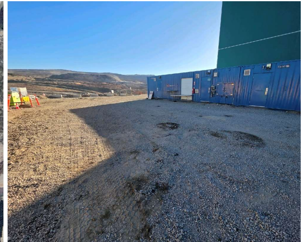
Photo 114471-1. Several spills to ground observed within a lined area at the Mobile Maintenance Yard. Opportunity for improvement issued to prevent tracking of hydrocarbon contamination out of lined area.
