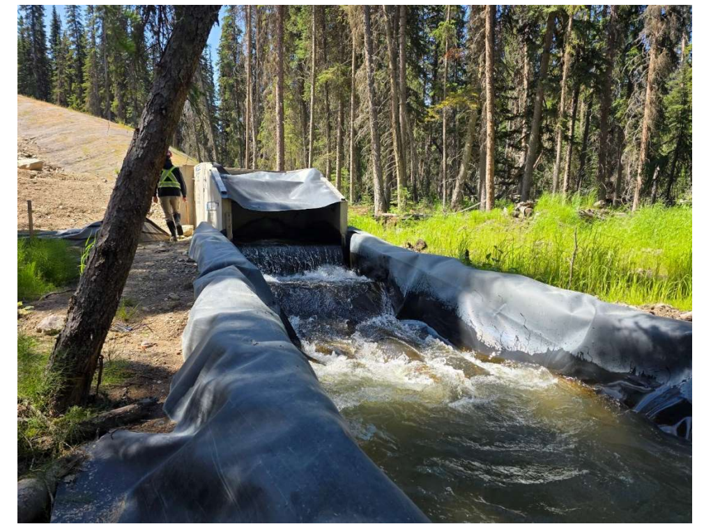
Photo 114070-3. Discharge from the Water Management Pond (WMP) outfall to Davidson Creek. Water is treated at the WMP treatment (clarifier) plant prior to discharge.
