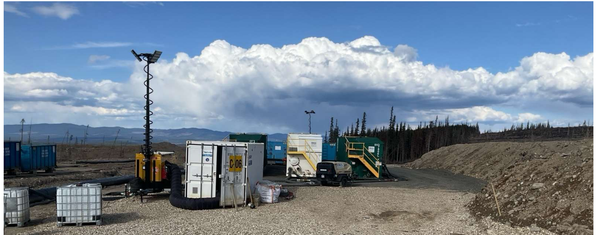
Photo 113697-2. Water treatment plant (clarifier) at the WMP to be utilized in the event water is required to be pumped to Davidson Creek.
