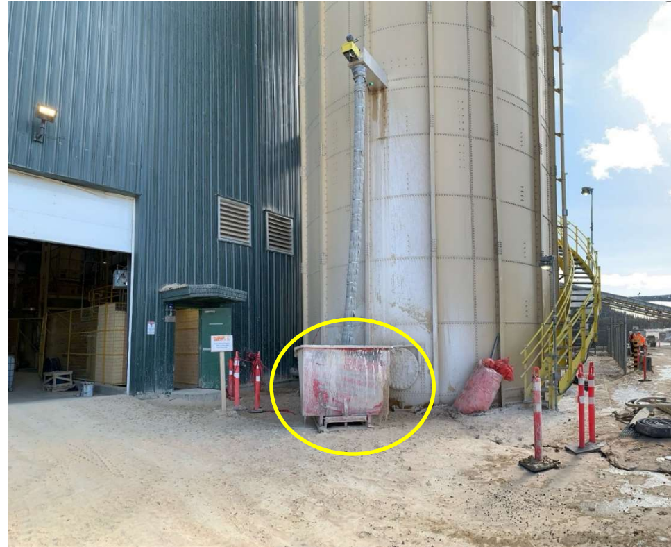
Photo 113331-3. Bin holding an unknown liquid adjacent to the lime silo at the Plant Site. Confirmed by BWG on March 22, 2025, to be water and grit/rock pieces from screen within silo.
