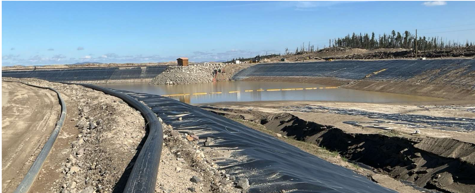
Photo 114313-7. Overview of the WMP. Decant tower currently not able to be used to send water to Plant Site due to sediment accumulation within the pump intakes.
