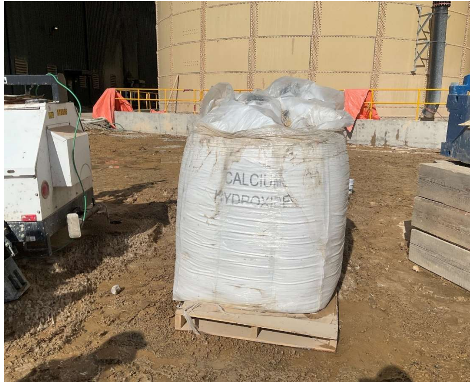
Photo 113342-1. Sack of calcium hydroxide (hazardous material) observed stored outside of secondary containment at the Plant Site.
