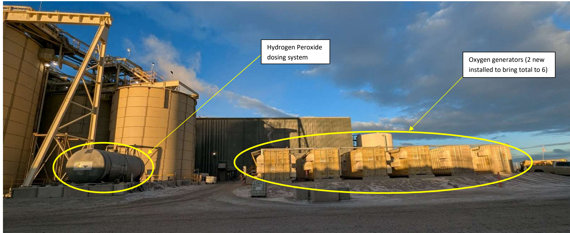
Photo 114725-5. Overview of two additional oxygen generators and hydrogen peroxide dosing system associated with improvements to the cyanide destruction circuit installed at the Plant Site.
