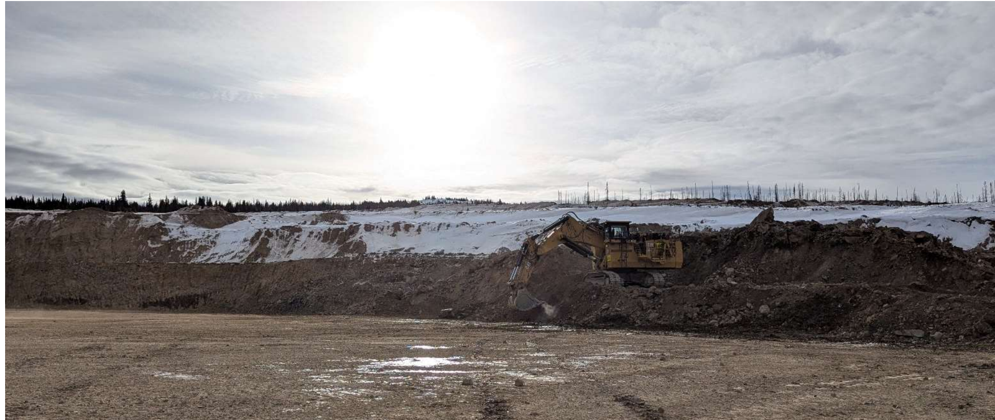
Photo 112957-2. Ongoing excavation within the open pit/ore body.
