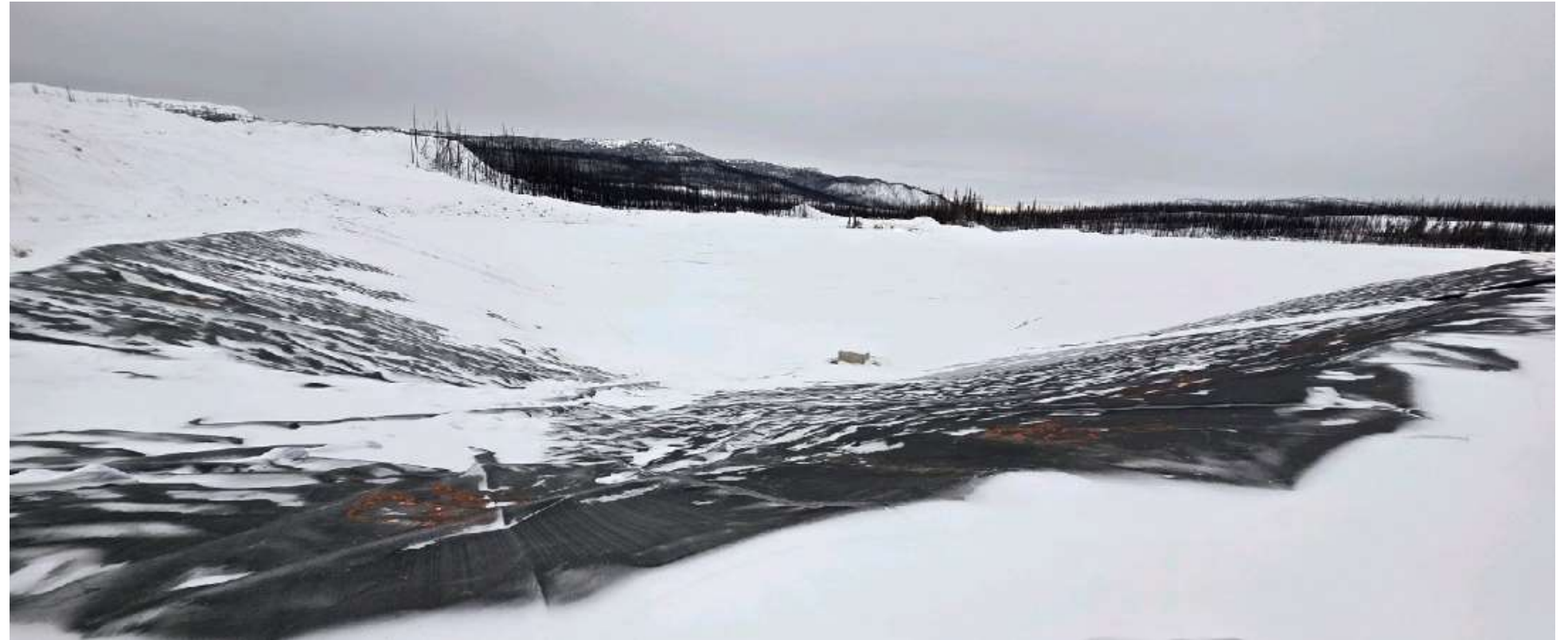
Photo 113124-2. Overview of the LGO stockpile pond following completion of liner installation.
