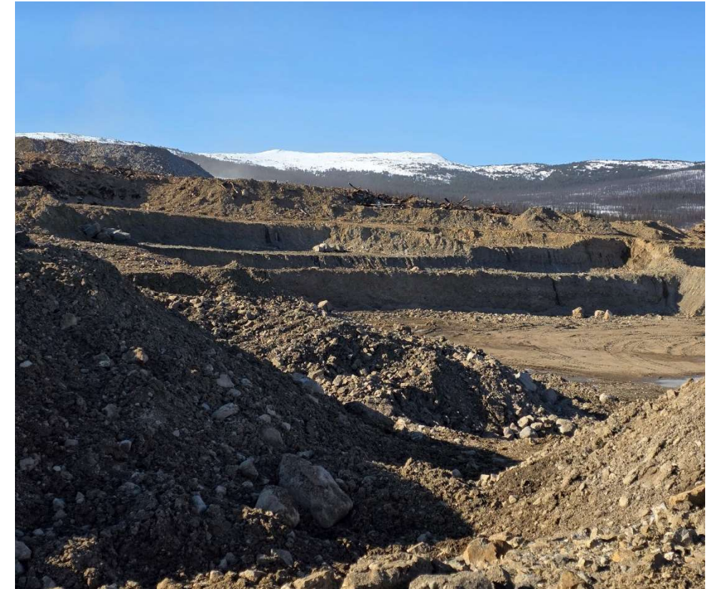
Photo 113556-7. Development of Borrow Pit 4 (source of zone s till material) adjacent to the LGO stockpile pad.
