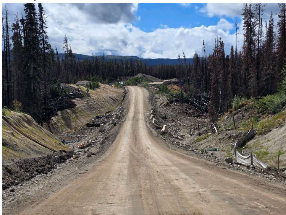
Photo 114199-4. Overview of former bridge crossing over Watercourse 636 at 9.5 km on the C-trail access road which has since been replaced with a culvert crossing.
