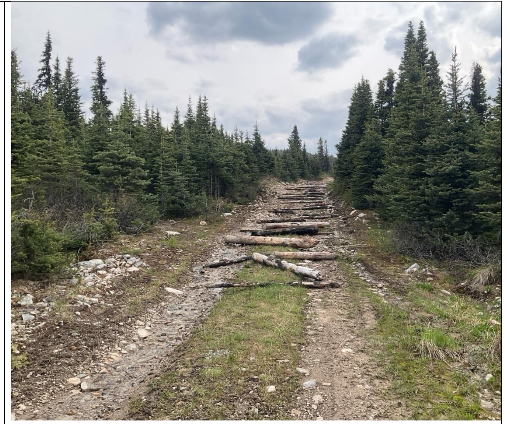
Photo113872-1 Large woody debris placed on Mt Davidson Exploration Road.
