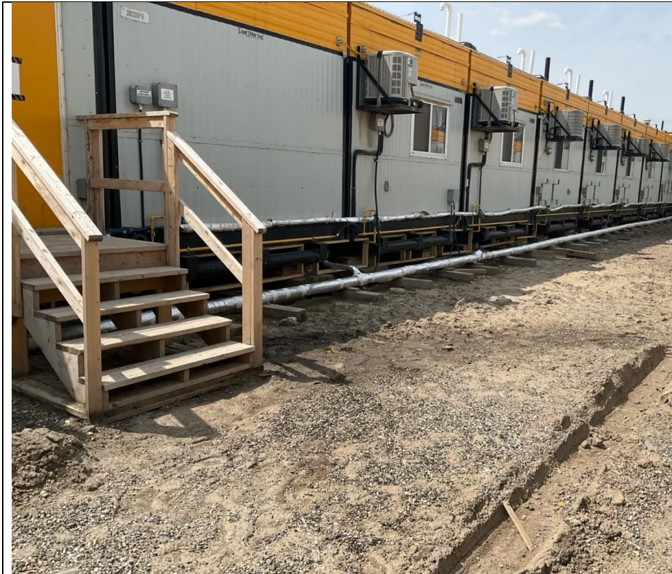
Photo113864-1 No skirting around the base of the kitchen trailers at the Operations Camp.
