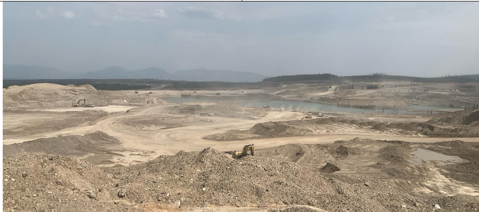
Photo 113871-1 Work continues within the Tailings Storage Facility.
