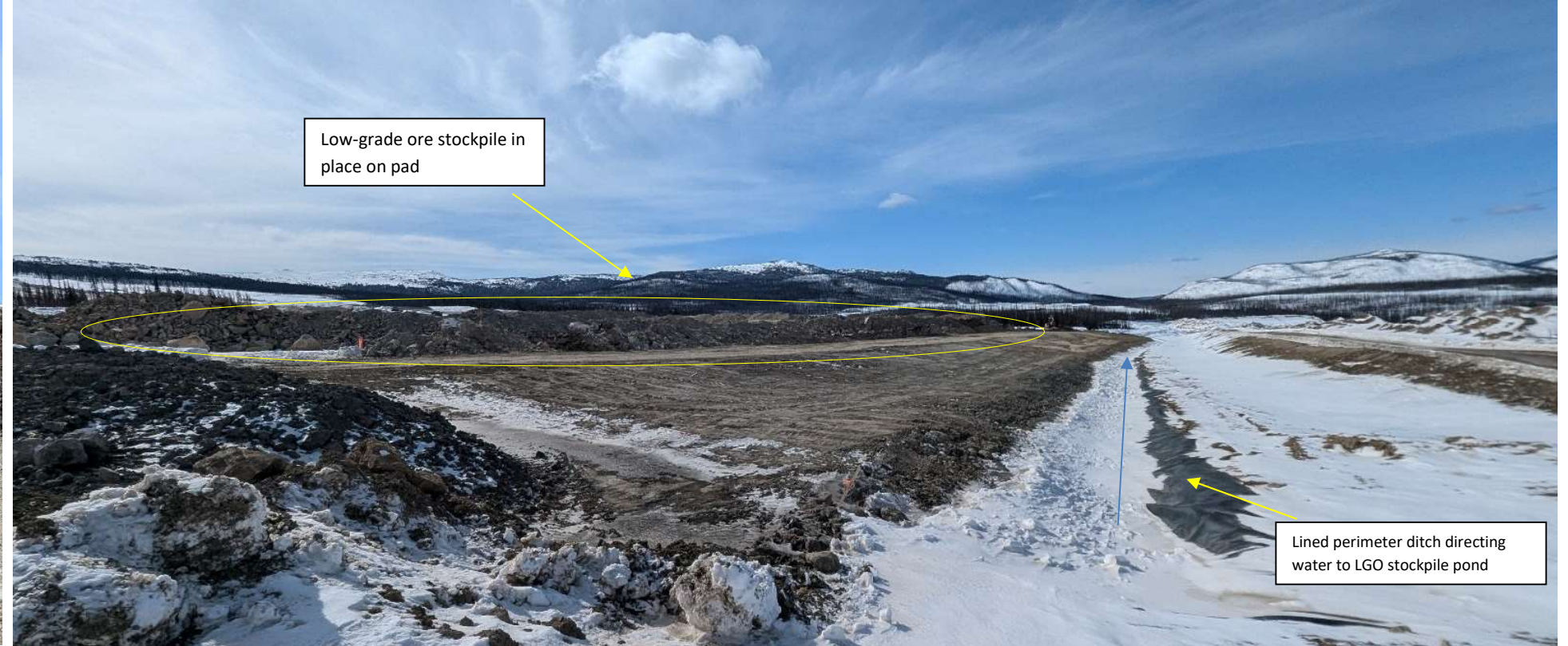
Photo 113327-3. Overview of completed portion of LGO stockpile pad.
