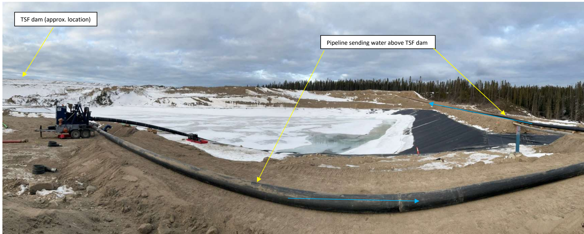
Photo 112946-4. Overview of water pooling on the upstream side of the Interim Environmental Control Dam (IECD). Water is being pumped (via pipeline) to the area upstream of the TSF dam.
