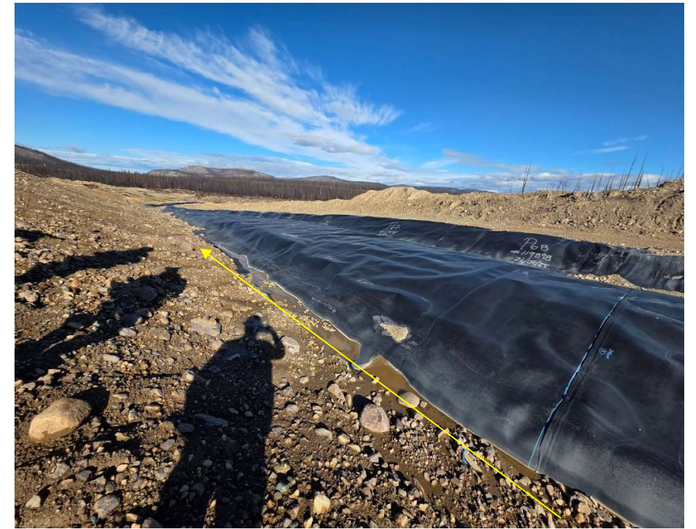
Photo 114219-4. Raised edge of LGO stockpile drainage ditch resulting in water flowing alongside channel as opposed to within it.
