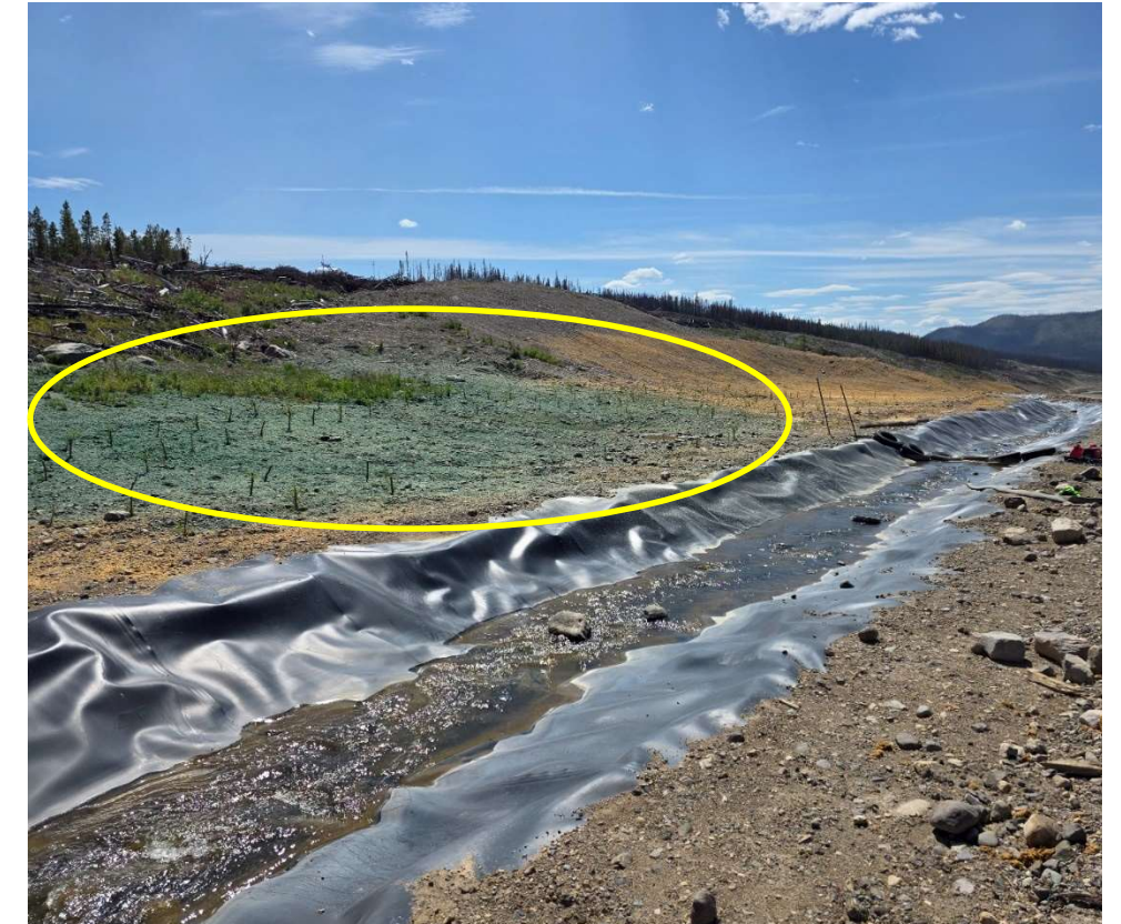
Photo 114074-2. Live staking and hydroseed application along the slopes adjacent to the upper extents of the Southern Collection Channel.
