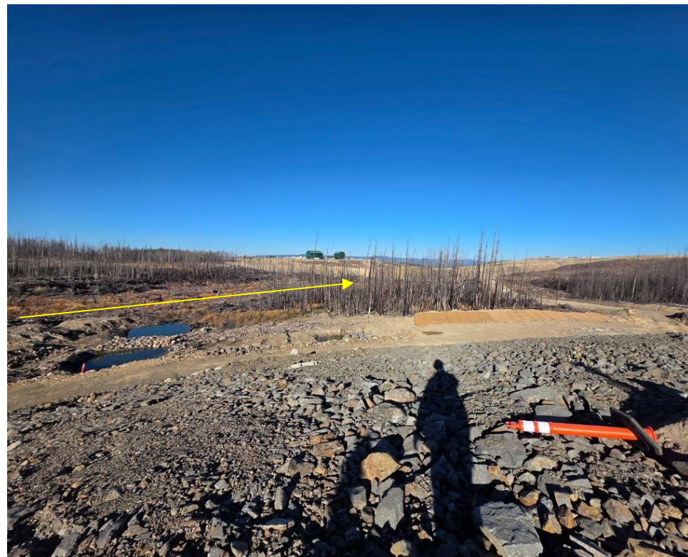
Photo 114470-15. Riprap armoring installed along slopes surrounding the LGO stockpile pond. Approximate pathway of Mine Creek indicated on photo for reference.
