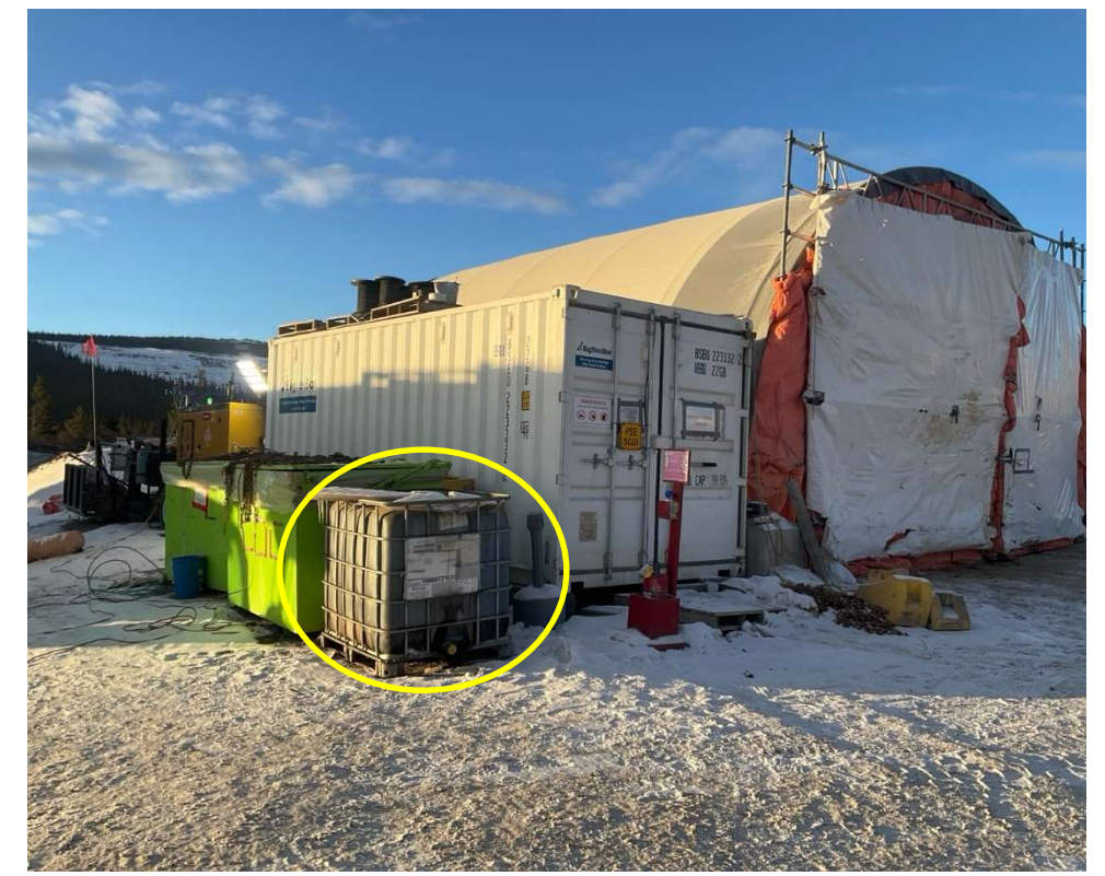
Photo 114728-3. Tote containing what appeared to be a hazardous substance (hydrocarbon contaminated water or waste oil) stored outside of secondary containment at the infrastructure laydown. BWG confirmed tote had been removed on December 4, 2025.
