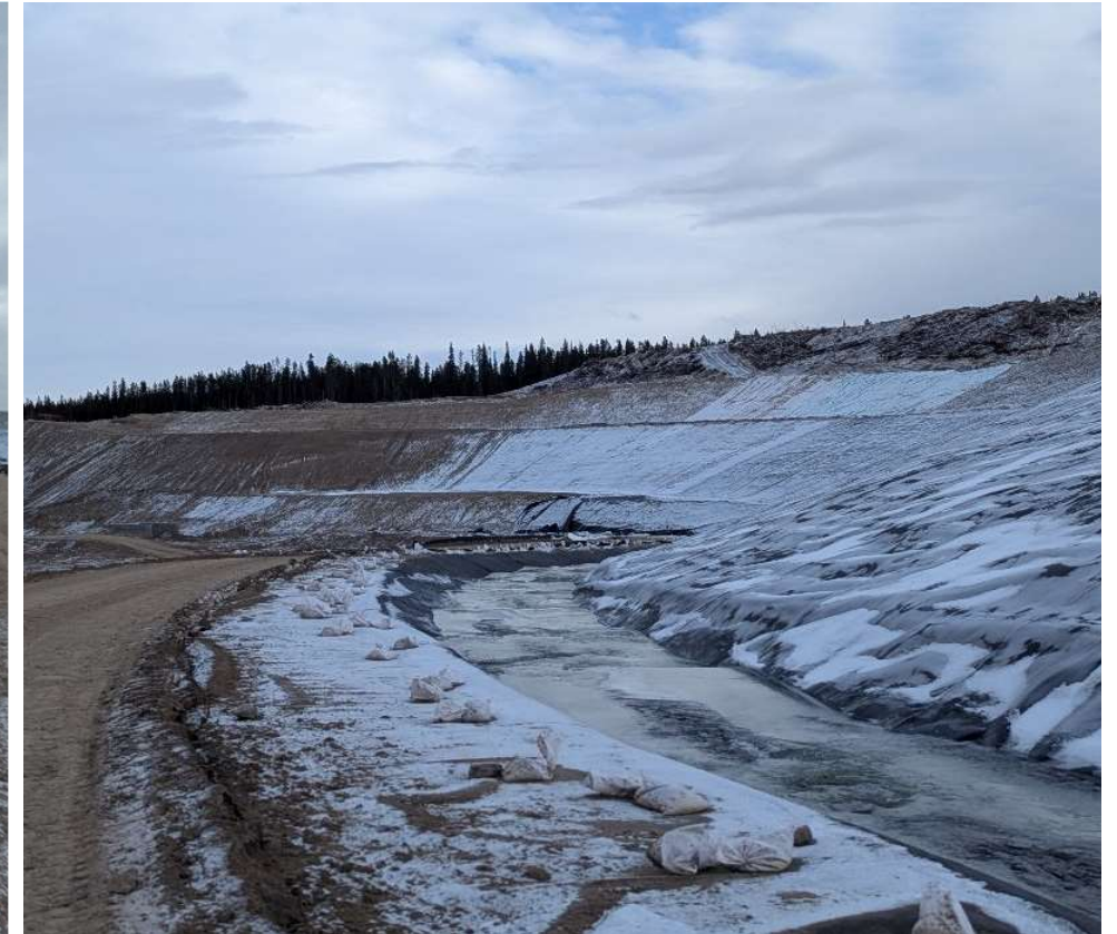
Photo 114702-2. Davidson Creek diversion along the base of the future Fresh Water Reservoir.
