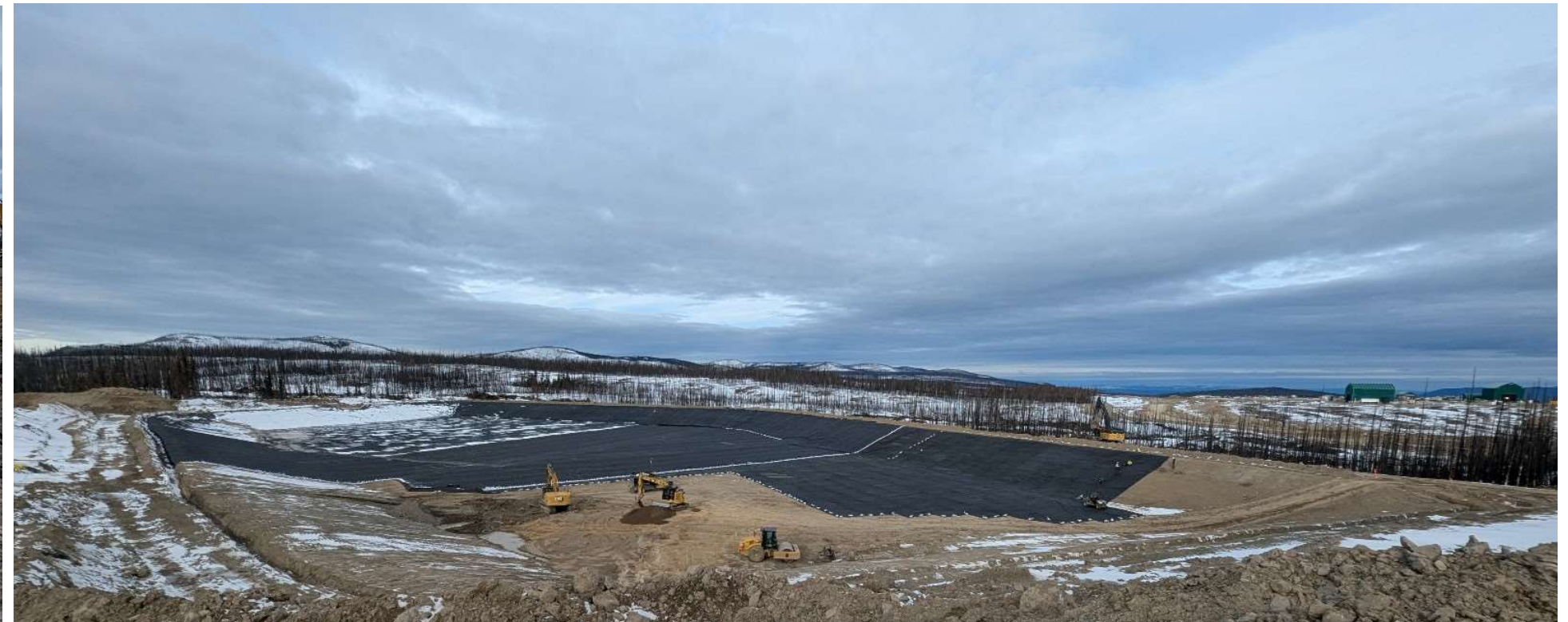
Photo 112954-4. Crews nearing completion of liner placement within the LGO stockpile pond.
