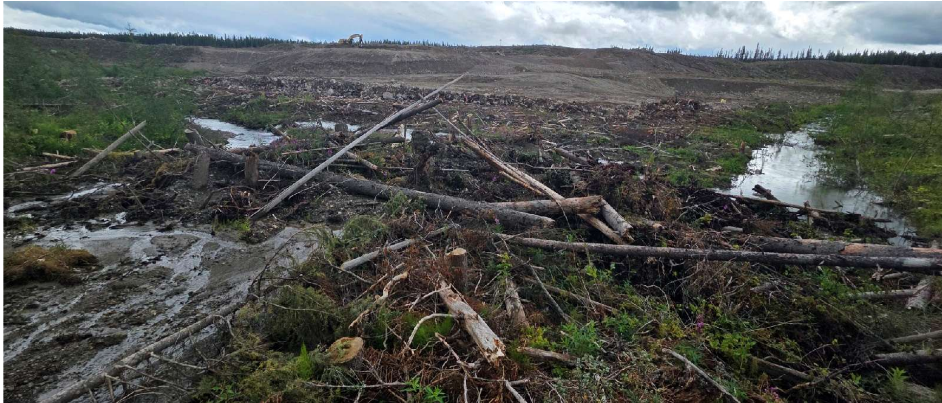
Photo 114201-7. Current state of Davidson Creek following slope failure within the Fresh Water Reservoir footprint that occurred on June 24, 2025. Current channel can be seen on high side of slide.
