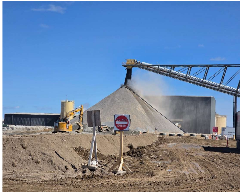
Photo 113515-1. Stockpile of high-grade ore at the drop point of the till conveyor. Stockpile height noted to be elevated in comparison to previous site visits, reducing drop height from conveyor.
