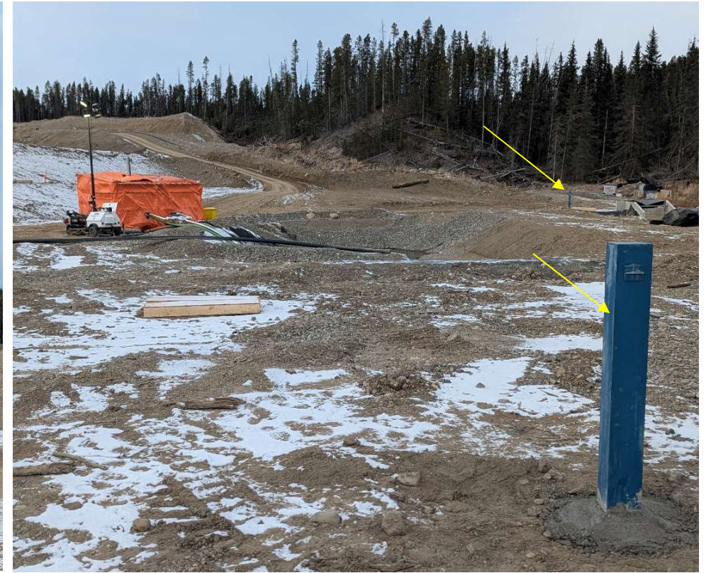
Photo 114712-4. New groundwater monitoring wells installed downstream of the IECD sump.
