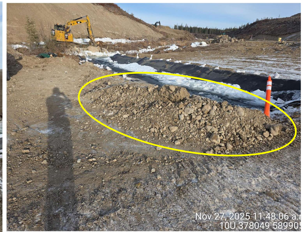
Photo 18. Material berm put in place at low spot identified along the Davidson Creek diversion channel within the Fresh Water Reservoir. Photograph provided by BWG on December 4, 2025.
