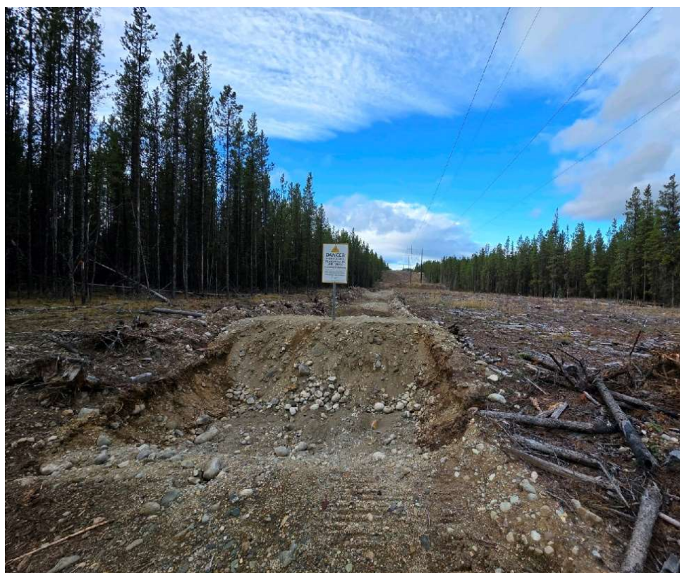
Photo 114490-4. Signage installed on top of an access road deactivation berm on the Transmission Line.
