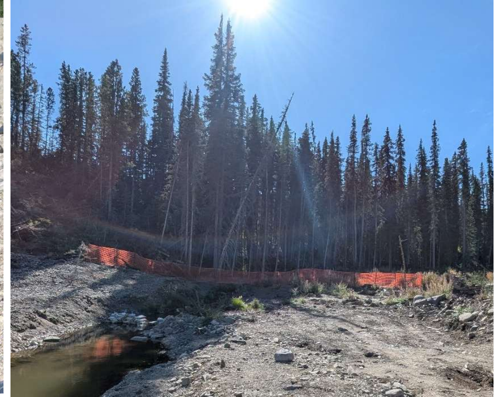
Photo 114313-3. Fencing installed at inlet to WMP to deter wildlife entry.
