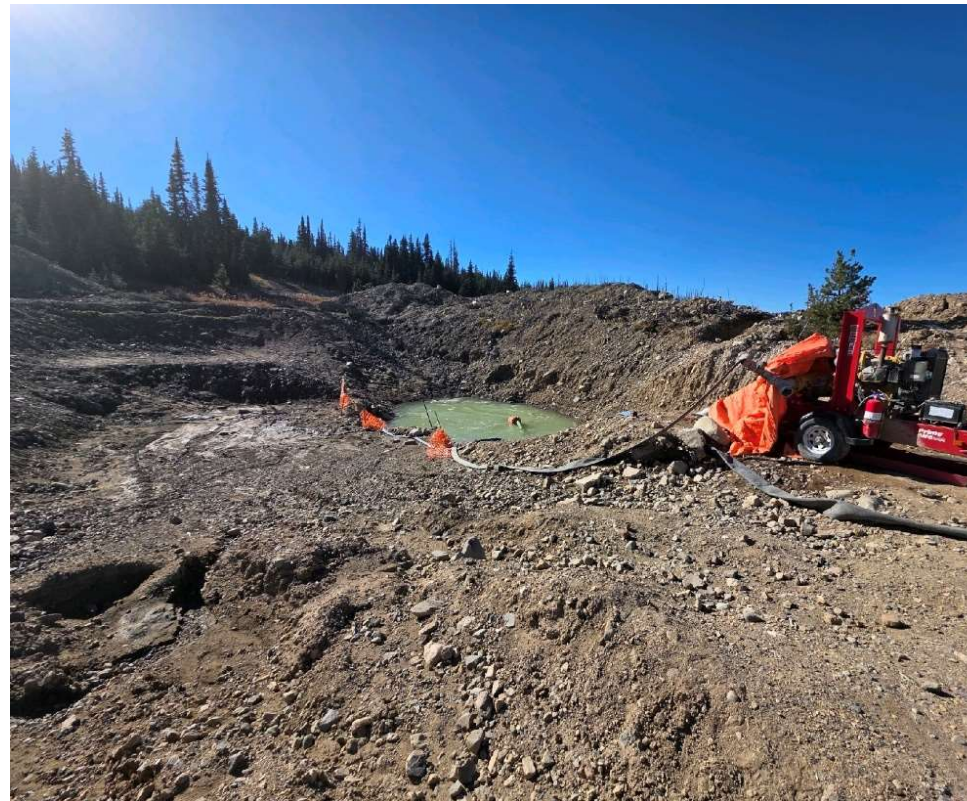
Photo 114451-1. Groundwater capture sump upslope of the open pit. Water from the sump is being pumped to a ditch line which sends the water towards the Mine Creek drainage (terminating within the WMP).
