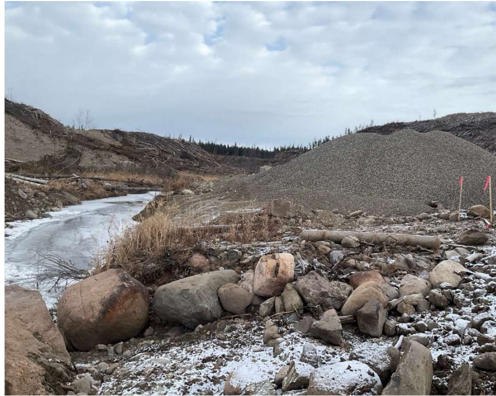
Photo 114706-1. Stockpile of aggregate (with some fines) located adjacent to Davidson Creek. IEM recommended this pile be removed to prevent sediment transport into Davidson Creek.
