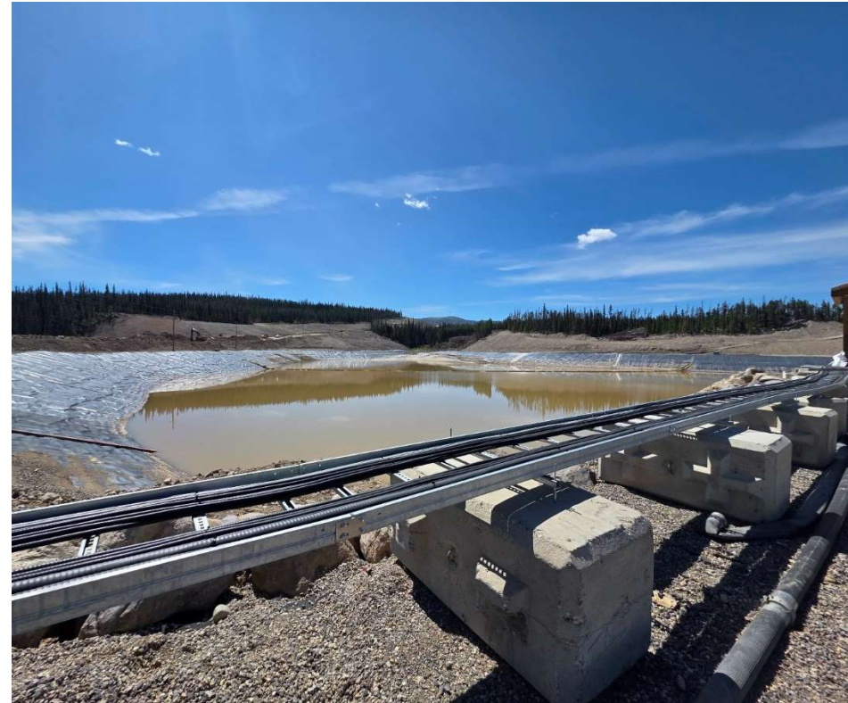
Photo 114071-4. Overview of turbid water within the water management pond.
