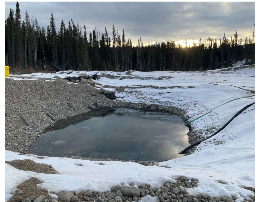
Photo 112946-1. Foundation drain (former groundwater collection point) downstream of the IECD that was previously discharging water to Davidson Creek, now has water pumped and discharged upstream of the IECD.
