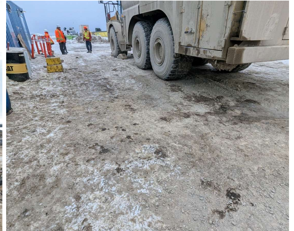
Photo 113349-5. Hydrocarbon stains (dark spots) on ground at the fuel and lube truck staging area at the Mobile Maintenance Yard.
