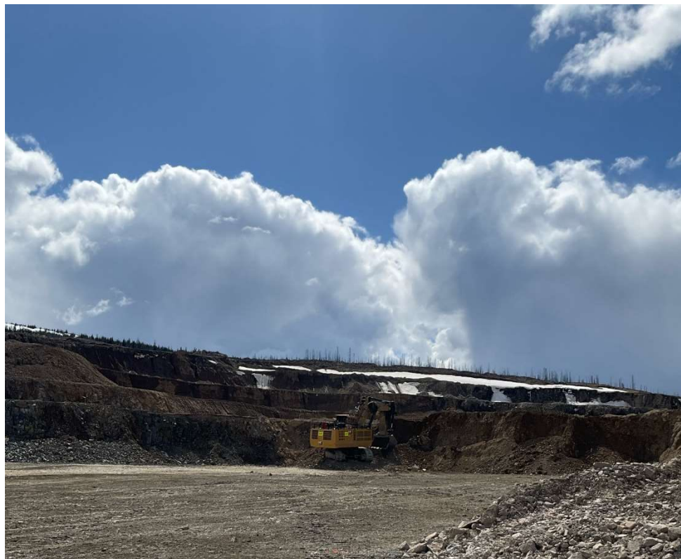
Photo 113686-1. Excavation and benching of slopes ongoing within the ore body/open pit.
