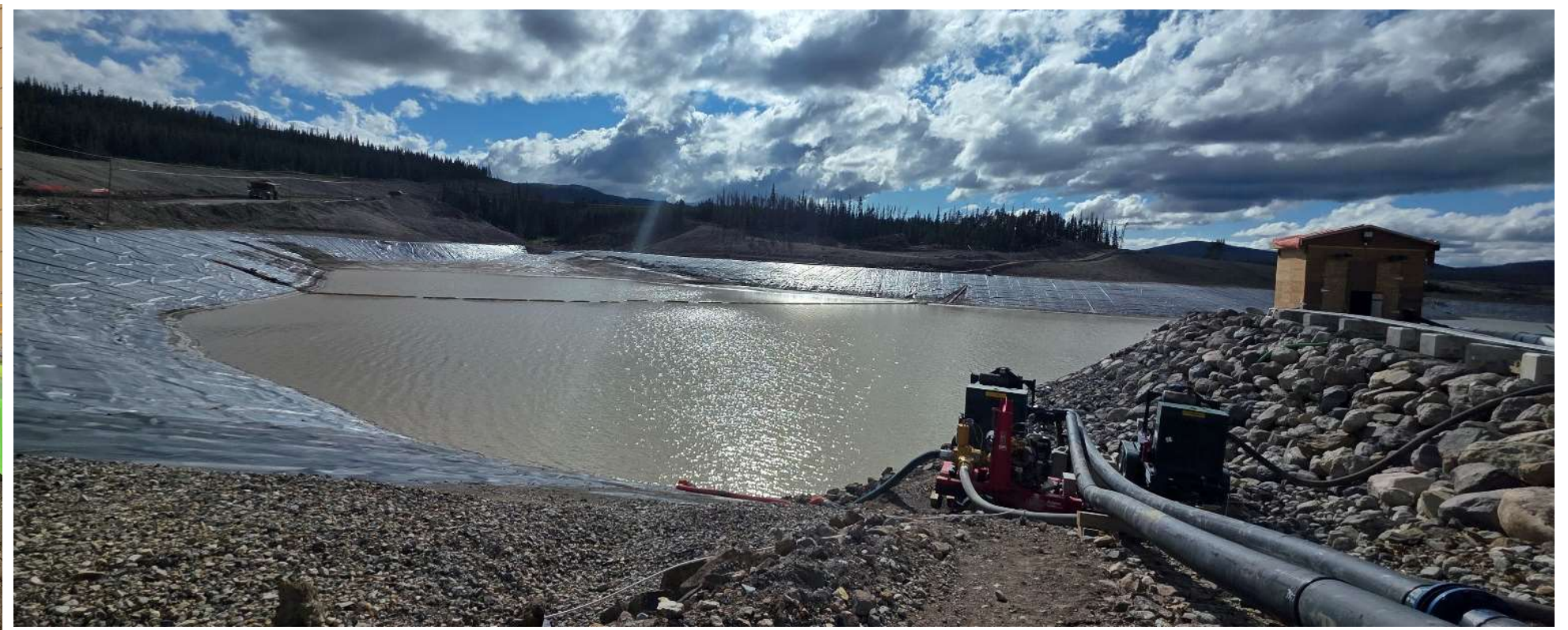
Photo 114205-4. Overview of low water level within the Water Management Pond.
