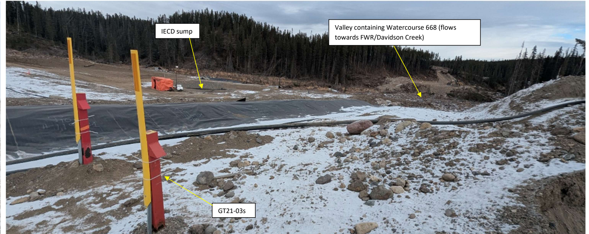
Photo 114712-3. Overview of the location of the groundwater collection point downstream of the IECD referred to as the 'IECD sump' where elevated levels of WAD Cyanide have been detected. Groundwater well GT21-03s and the valley containing Watercourse 668 (flowing towards the FWR) labelled for spatial reference.
