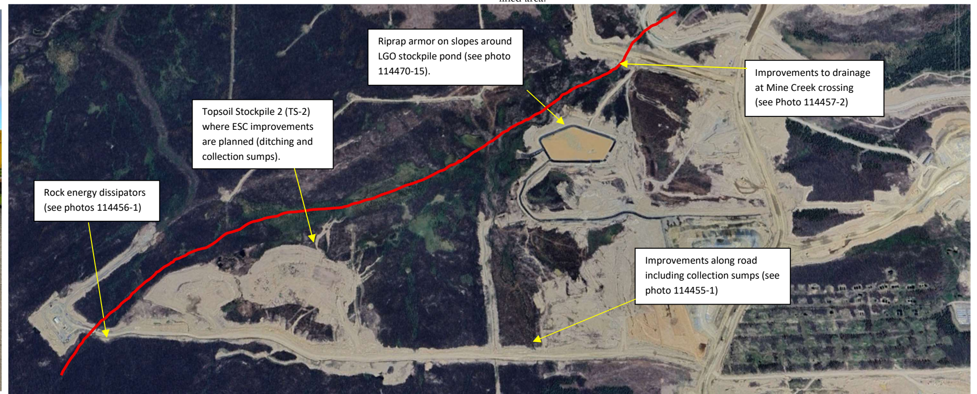
Photo 5. Summary of locations of ESC improvements implemented within the Mine Creek drainage. Note that this may not include all improvements made to date. Additional detail can be seen in subsequent photos referenced. Generalized pathway of Mine Creek sketched onto photo for reference (in red).
