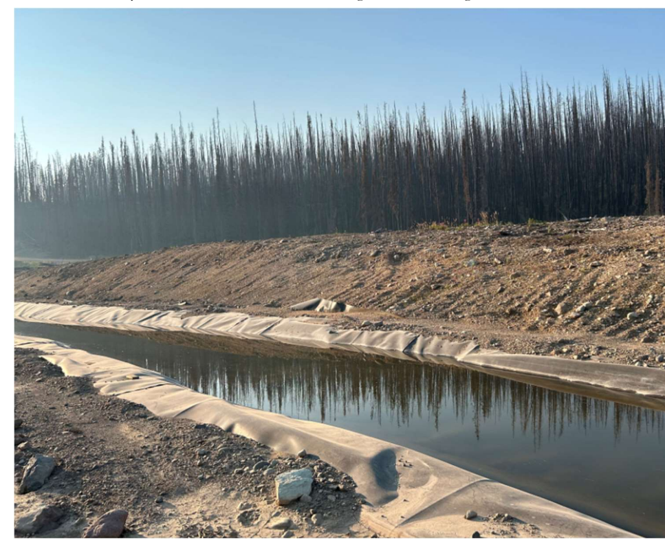
Photo 4. Confirmation of removal of sediment accumulation from the South Collection Channel. Photograph provided by BWG on September 8, 2025.
