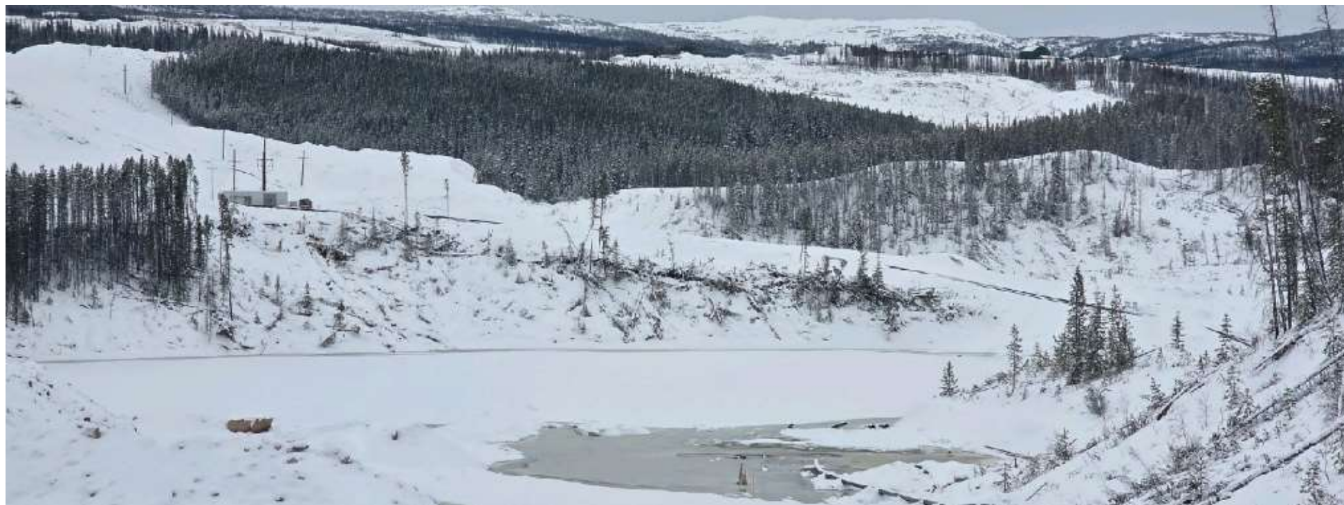
Photo 113132-5. Water accumulation upstream of the DCDS. Barge pump in place sending water to plant site upstream of photo (out of frame and unable to be observed due to access constraints).
