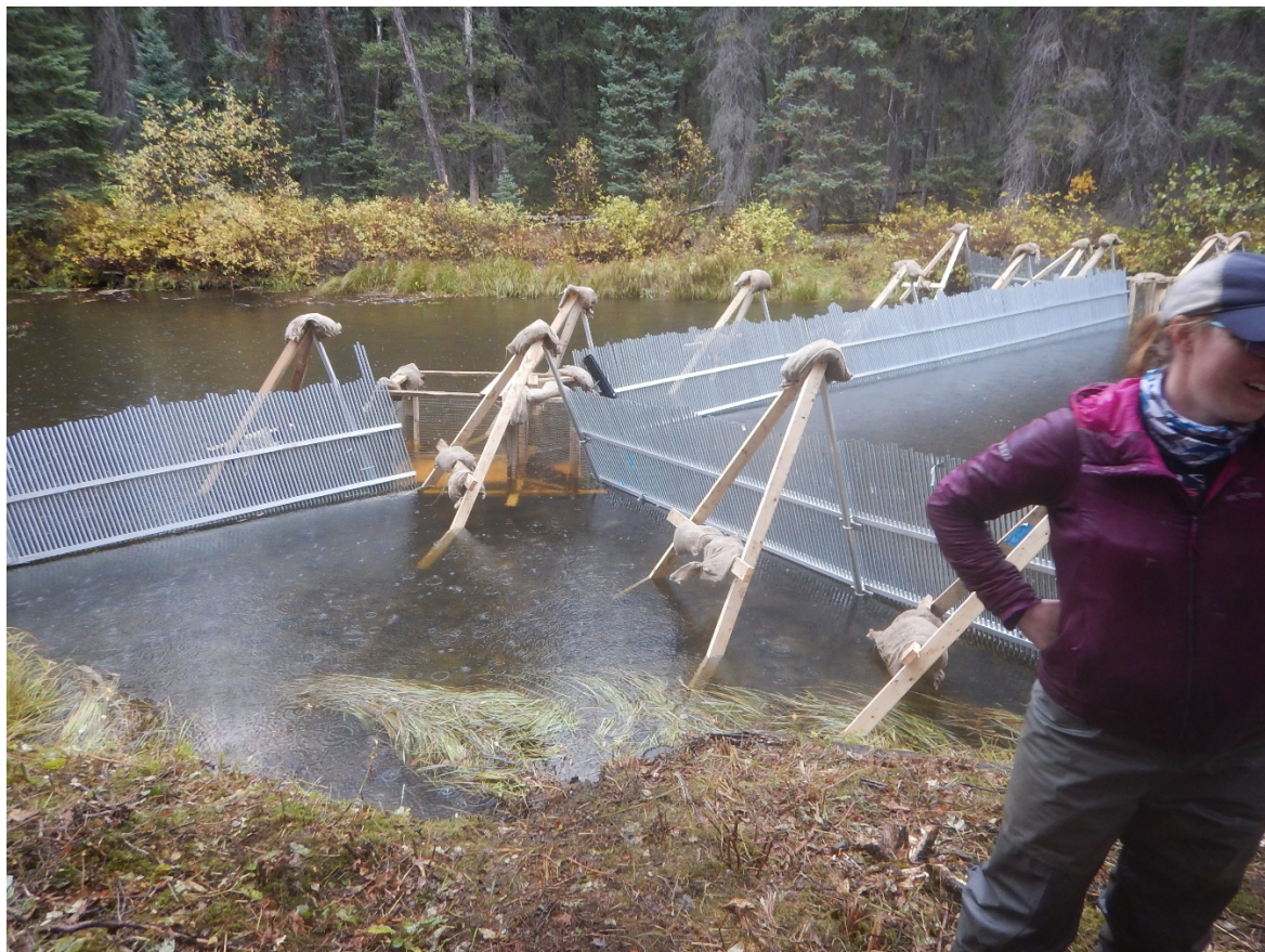
Figure 9 Conduit weir built in Philip Creek in fall 2020 for Thompson Creek Metals Company
