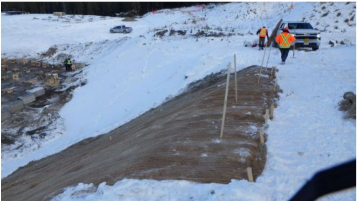
Figure 4 - Erosion control blankets installed on slopes adjacent to the temporary camp
