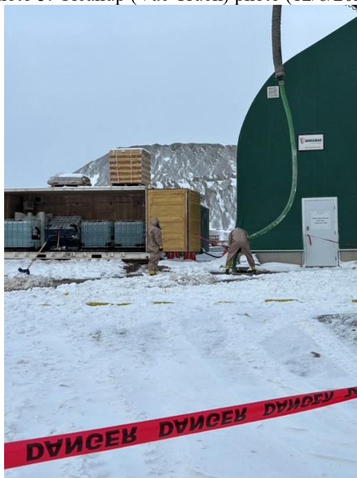
Photo 6: Cleanup (Vac Truck) photo (12/6/2025)
