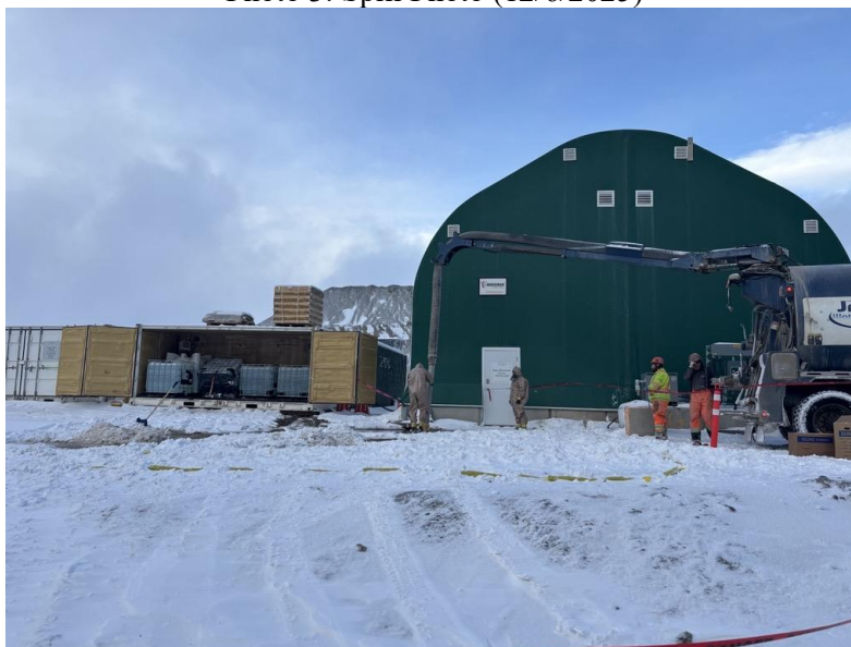
Photo 4: Cleanup (Vac Truck) photo (12/6/2025)
