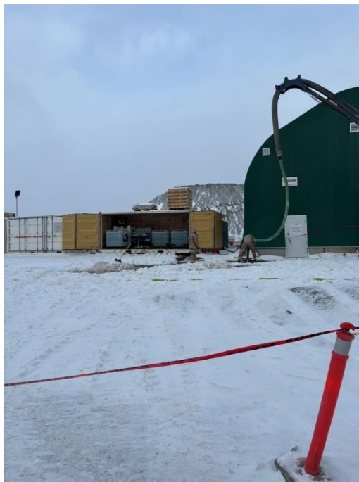
Photo 5: Cleanup (Vac Truck) photo (12/6/2025)
