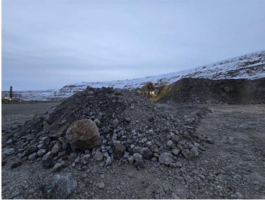
Photo 5: Contaminated material pile prior to removal
